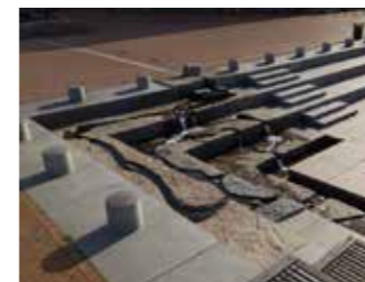
SuDS incorporated into hard landscaping as feature elements of the public realm
