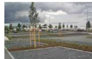
Permeable paving incorporated into parking areas
