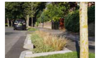
Nottingham's Ribblesdale Road - rain garden SuDS retrofit
